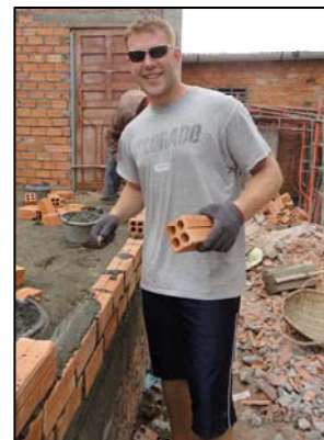
Jameson mastering brick laying
