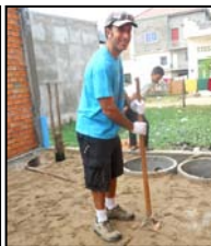
Craig leveling the floor
