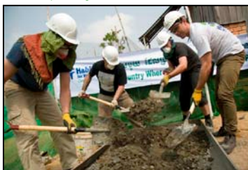
Team EJAF mixing cement
