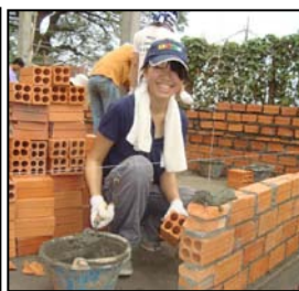
Sayo laying bricks
