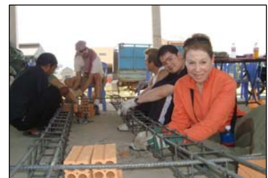
Enjoy tying the steel bars
