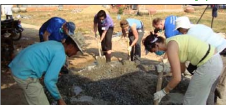
Mixing concrete as a team
