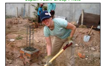
Ashleigh working on foundation
