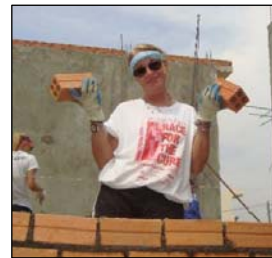
Bricklaying at its best!
