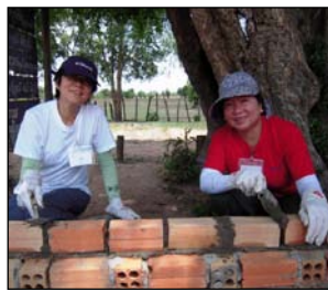
Starting the brick laying
