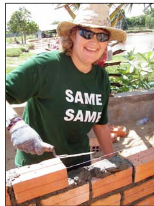
Having fun laying bricks
