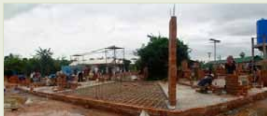
Community Center foundation building in progress
