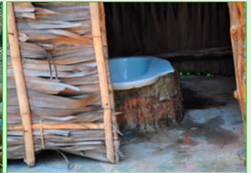
A completed creative toilet
