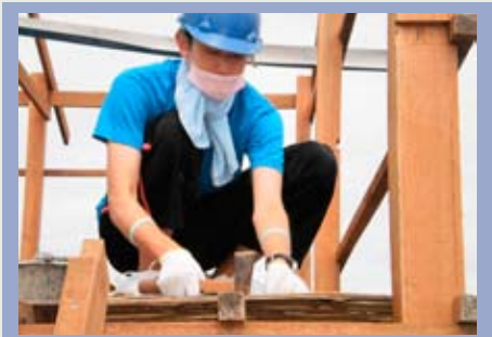
Nailing the wooden floor
