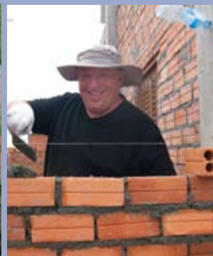
comfortable laying bricks
